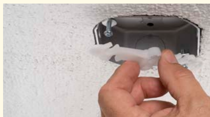
1 Easy installation. Attach the bracket to the box with #8 or #10 screws. Back the screws out enough to slip the bracket on.
