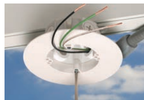
3 Attach medallion to box with supplied #8 x 1-1/4" screws.
