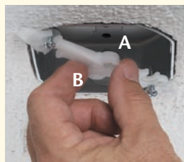
2 Use the bracket opening that works with the ceiling condition: 'A' for flat ceilings, 'B' for uneven or textured ceilings
