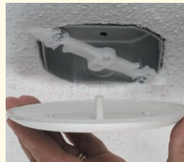
3 On flat ceilings, push threaded post into the 'A' opening to seat the cover. On textured or uneven ceilings, thread the post into the 'B' opening until tight.
