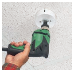
1 Cut hole in the ceiling with 4" hole saw.
