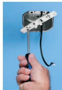
1 Attach SC5 bracket to box.
