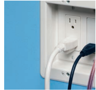
3 Install devices, then the wall plates.
