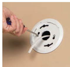
3 Install mounting plate per manufacturer's instructions
