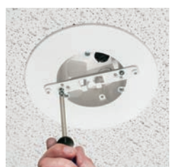
5 Install mounting bracket to inside of box.
