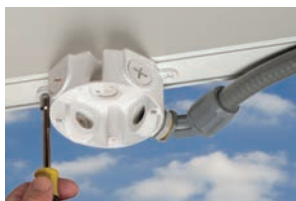
1 Install fitting with conduit. Seal unused openings with supplied plugs. Mount box to structural member.
