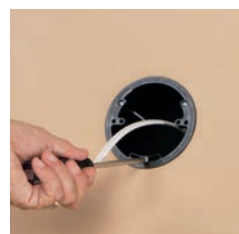
2 Pull cable and tighten mounting wing screws to hold bracket secure
